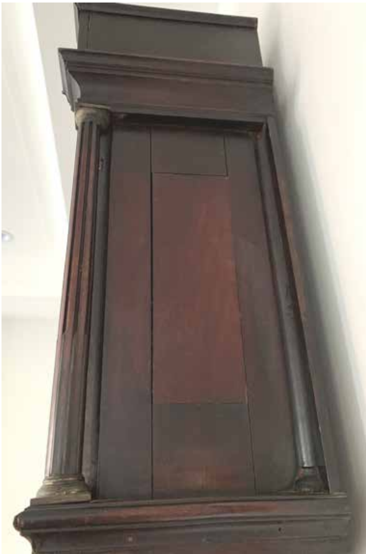
Figure 6. The sides of the hood have wooden infill pieces where originally would have been frets in brass or wood or possibly glass windows.
